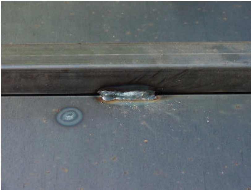
Figure 29 – Welds should be approximately 1" long.
